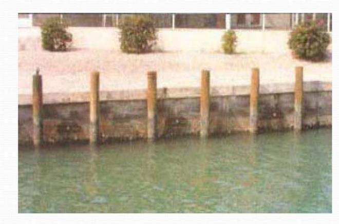
Wood pilings are also used for stabilization. This seawall also has galvanized steel channels just above water level which are anchored to deadmen in the same manner as a waler
