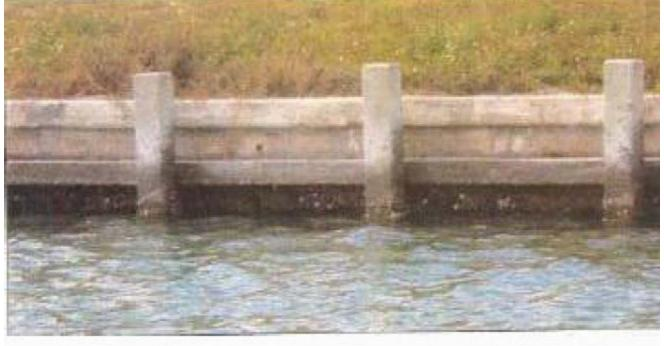
This seawall has a waler plus pilings driven into the canal bottom for extra support. The pilings help stabilize the wall to keep the toe from moving out.
