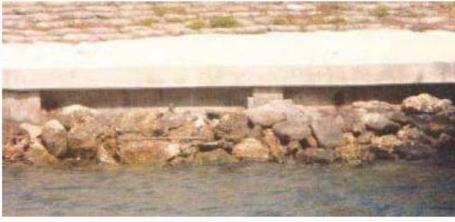
Rip-Rap (stone piled against the seawall) is particularly useful in areas of high tidal velocity to keep berm sand from washing away. The negative of Rip-Rap is that it extends out from the wall and can hamper boat docking unless there is a dock extending out over the Rip-Rap.
