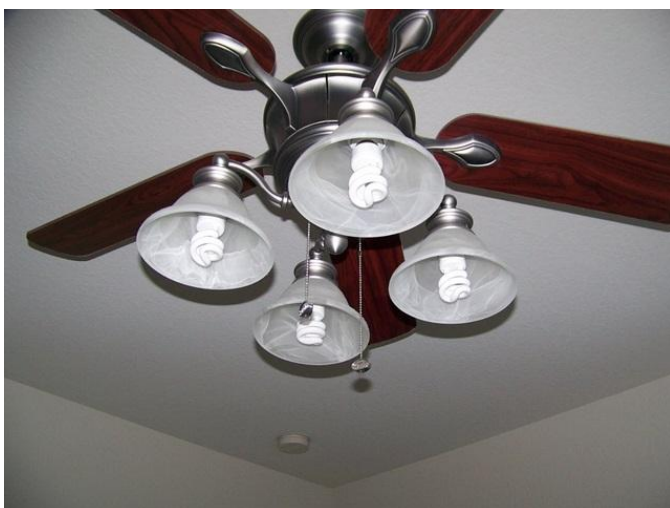
Picture #25 Family Room Ceiling
