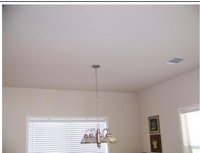
Picture #21 Dining Room Ceiling
