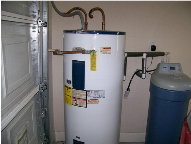
Picture #63 Hot Water Heater
