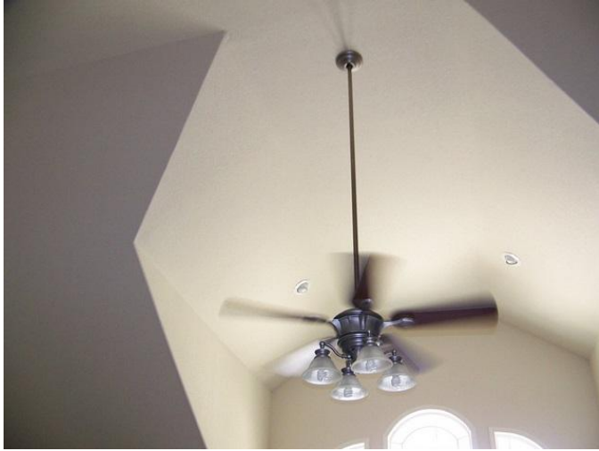
Picture #15 Living Room Ceiling
