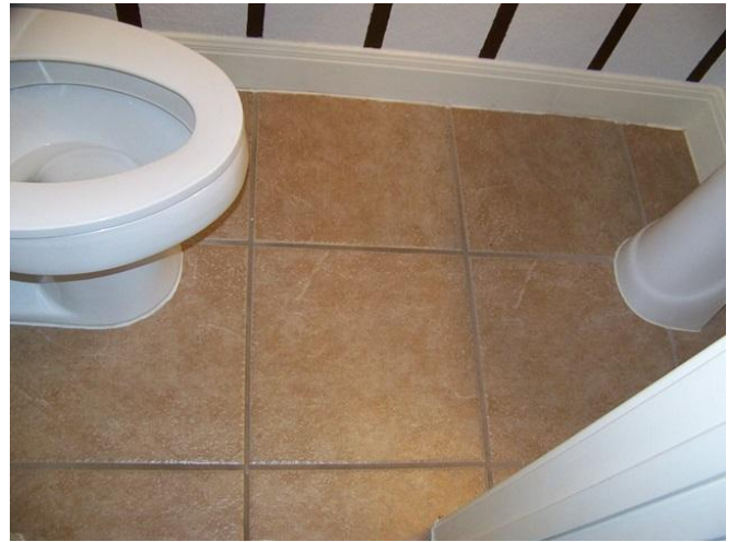
Picture # 52 Bathroom Floor
