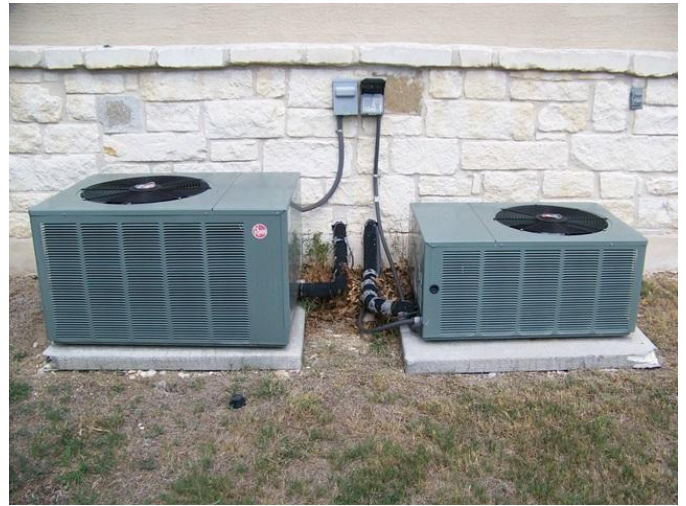
Picture #7 Picture of AC Unit
