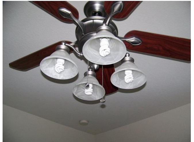
Picture # 50 Ceiling (Fan/Smoke Detector)
