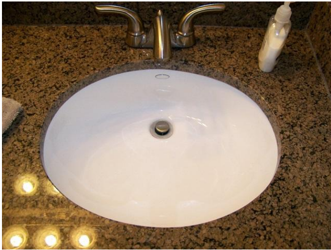
Picture #57 Sink and Faucets
