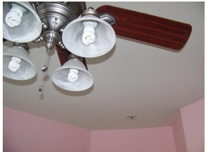
Picture # 46 Ceiling (Fan/Smoke Detector)
