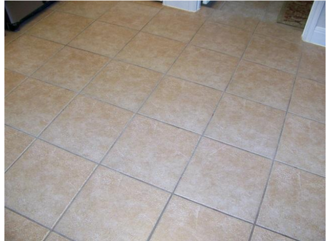
Picture # 30 Kitchen Floor
