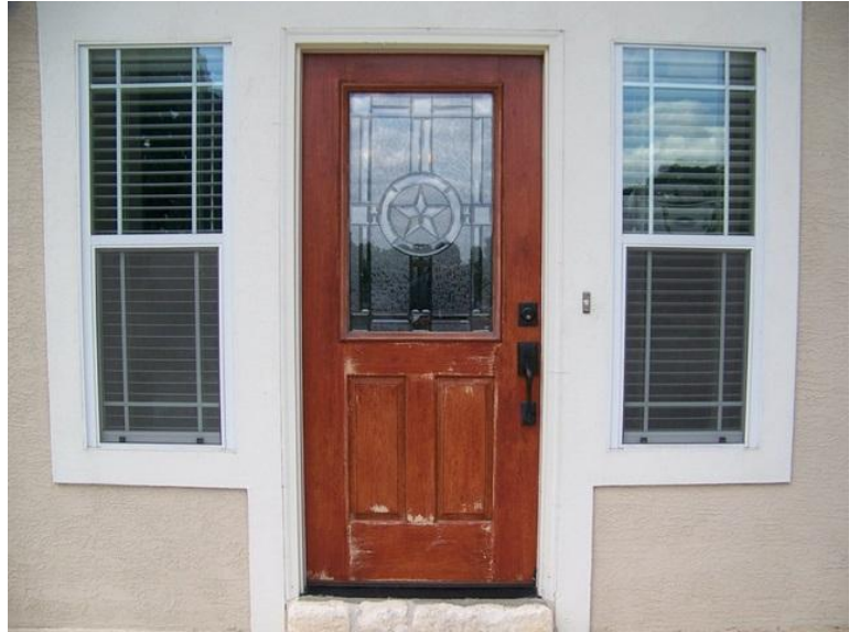
Picture #10 Front Door including casing.
