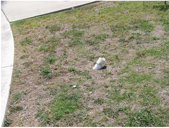
Picture #67 Trip Hazards
