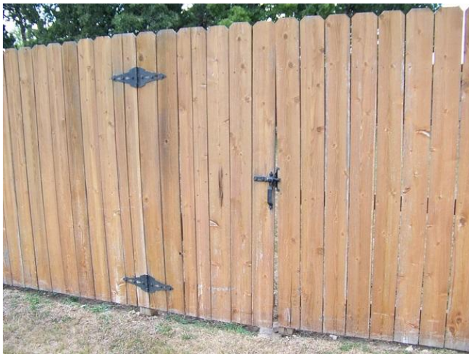
Picture #8 Picture of Fence and Gate
