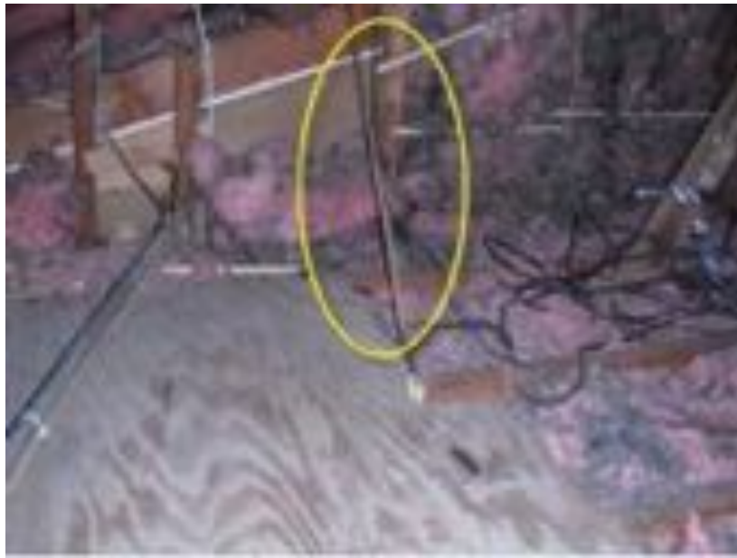
Gas lines and ROMEX cables must not be run together but separated to prevent contact
