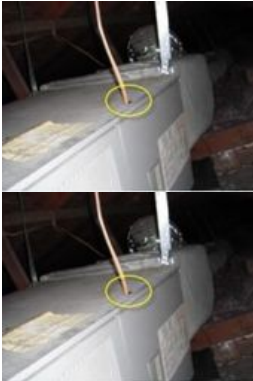
Only metal covers should be used on switch boxes, junction boxes and outlets in an attic
