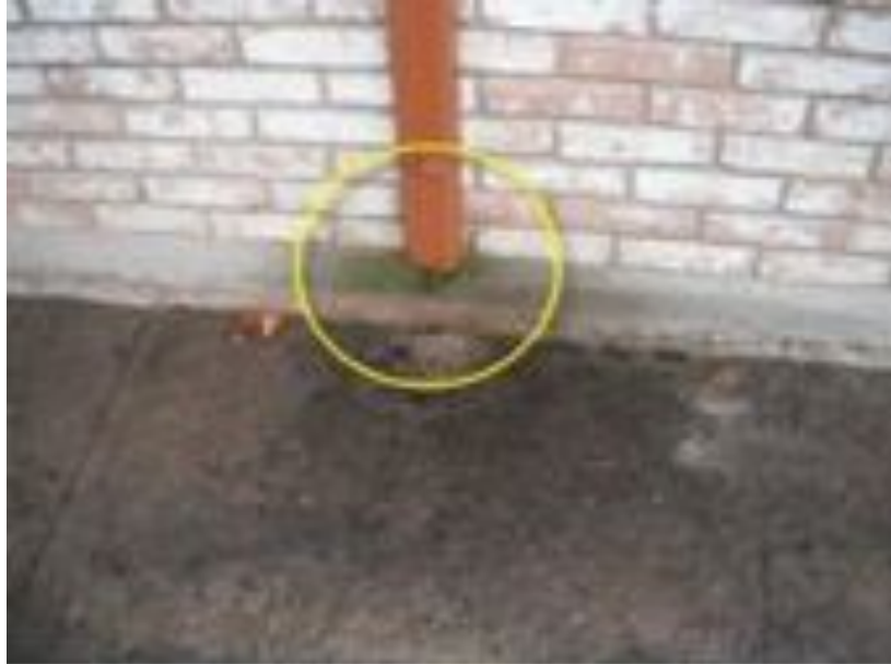
Clear gutters at front elevation
