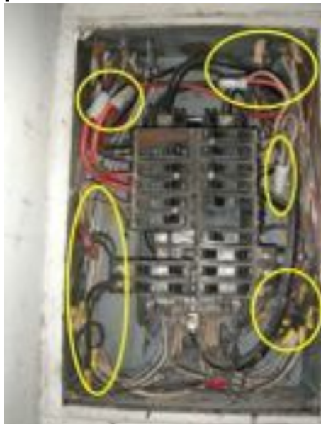
Over heating circuits in panel
