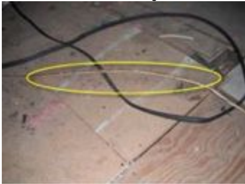
Protect all ROMEX cables running over service boards
