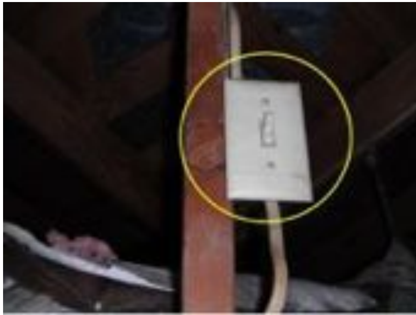
Protect all ROMEX cables running over service boards
