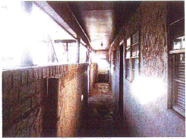
First Floor Walkway
