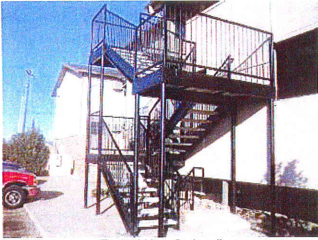
Typical New Stairwell
