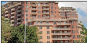
METROPOLITAN PLACE PHASE II : Downtown, 2bdrm, 1 ba & 1040 sq ft, southern exposure, new condo on 5th floor, stainless appliances. Ext 786
