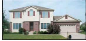
2797 SUNFLOWER DR, FITCHBURG : Sharp 4 bdrm, 3.5 bath in Swan Creek with higher end finishes and finished LL. 2500+ sq ft. Ext 856
